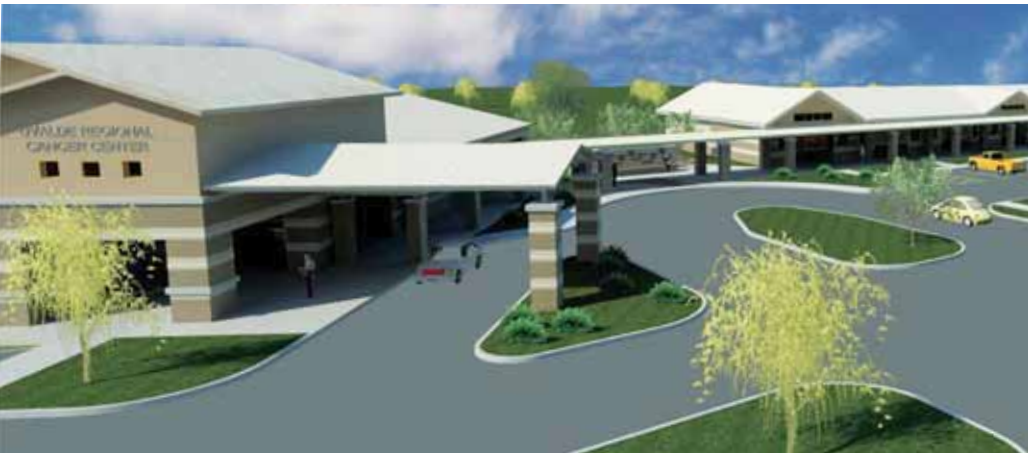
Groundbreaking: Wade Carpenter Photography; Rendering: O'Connell Robertson
